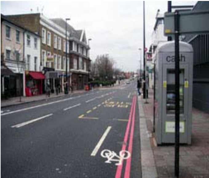
Battersea Bridge Road
