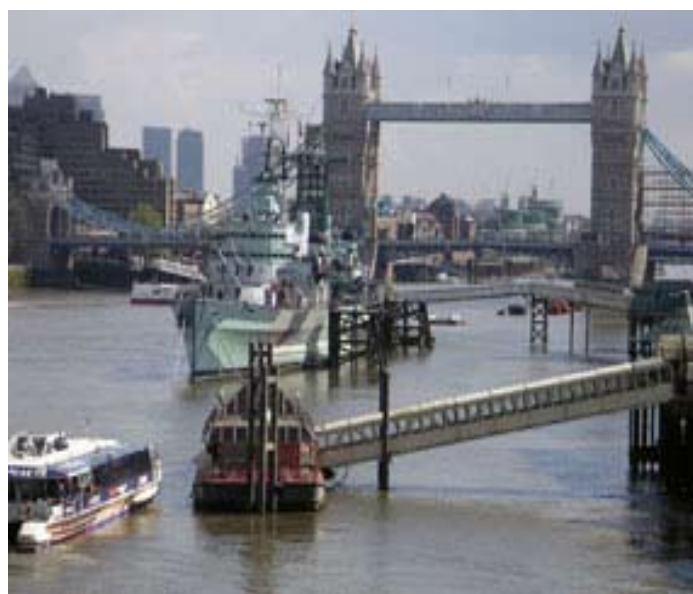
Tower Bridge - HMS Belfast
